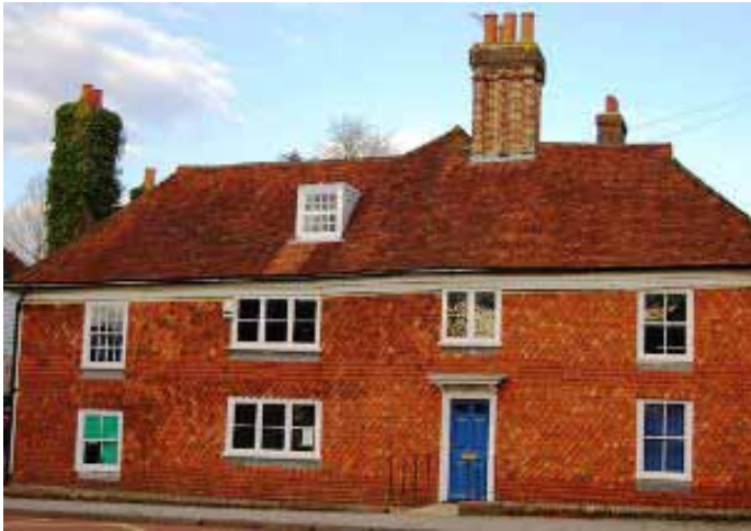
Ornamental shapes on a tile hung house in Robertsbridge © N Chadwick, Geograph (CCL)
