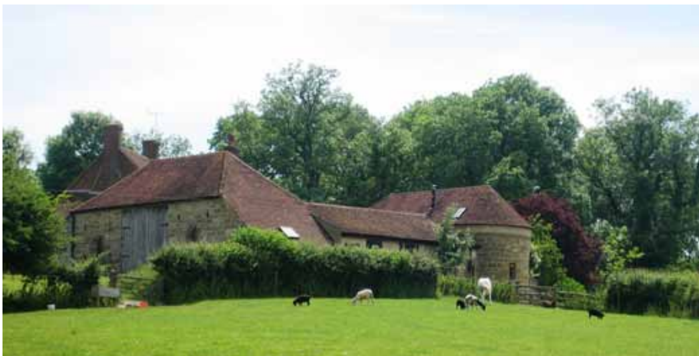
Typical architectural features of the Wealden landscape: hung tiles, a stone barn, catslide roof and round granary © Tim Locke
